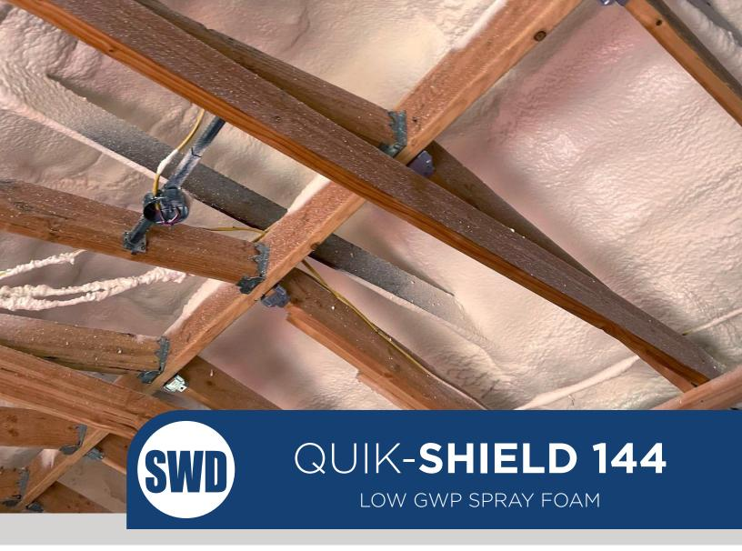
QUIK-SHIELD 144 is free of Hydrofluorocarbons (HFCs) meeting Global Warming Potential initiatives. With an R-Value of 7.5 per inch QUIK-SHIELD 144 offers superior performance and serves as an air barrier ideal for both residential (IRC) and commercial (IBC) construction.
