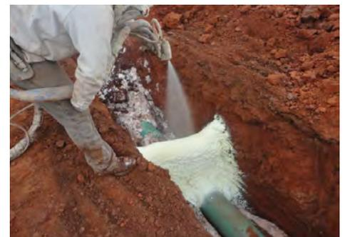
installation stability, high compressive strength, excellent adhesion, and because it is engineered for low exothermic reaction.
