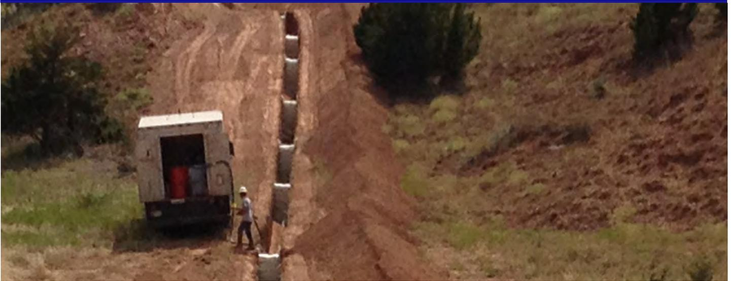
The use of Spray Polyurethane Foam in geotechnical applications for the oil and gas industry has proven to have a number of advantages and has grown in popularity in recent years.
