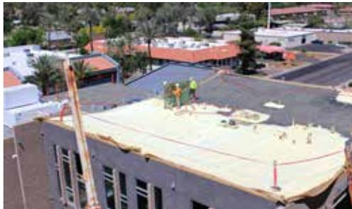
*A crane was used to bring the poly-iso boards up to the roof, where they were fastened down and covered with spray foam. The spray foam creates a monolithic seal to prevent thermal bridging from the fasteners.*
