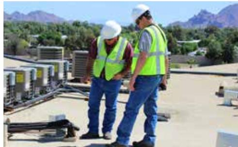
*Because the spray foam is self-flashing, it is ideal for sealing the roof penetrations made by other trades when installing conduits, vents, and HVAC lines.*
